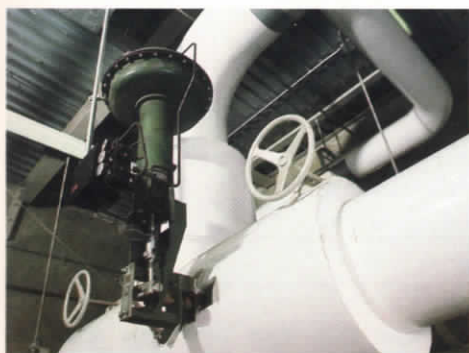
The large pipes carry water and the small ones carry ammonia to and from the steel ice-bank tanks. At a juncture of pipes (left), water leaving the ice bank is mixed with warmer water to raise its temperature to 42 degrees Fahrenheit before it is circulated to the research offices and laboratories.
