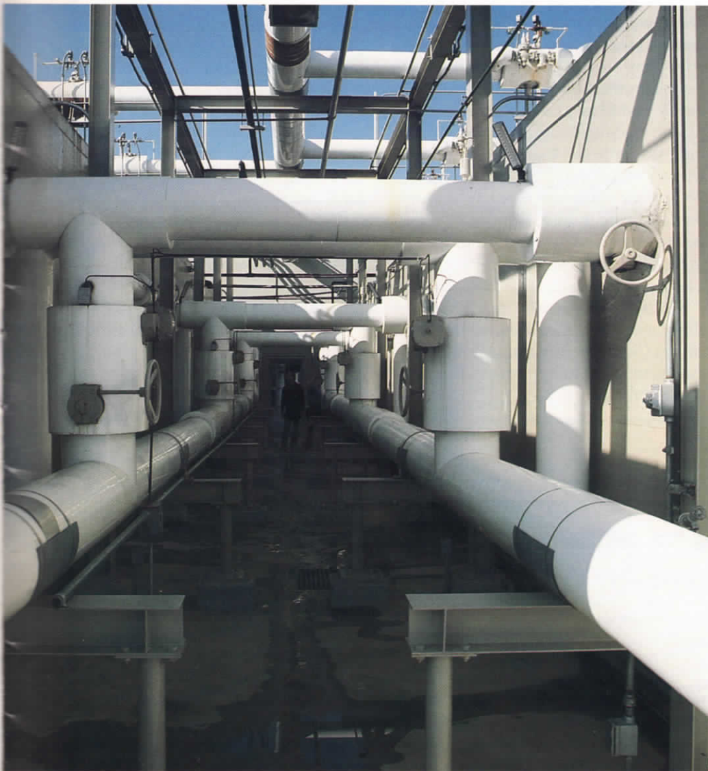
The large pipes carry water and the small ones carry ammonia to and from the steel ice-bank tanks. At a juncture of pipes (left), water leaving the ice bank is mixed with warmer water to raise its temperature to 42 degrees Fahrenheit before it is circulated to the research offices and laboratories.
