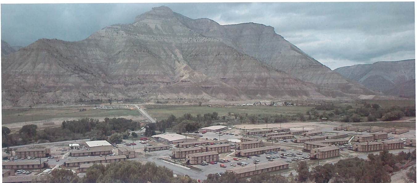
Housing complex will accommodate 900 single-status construction workers.
